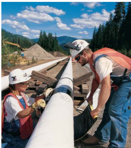
Company pipelines employ ConocoPhillips Specialty Products drag reducer technology, resulting in the ability to move more barrels of product with less energy. In addition, the drag reducer allows the pipelines to be operated at a lower pressure, reducing energy costs.
