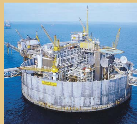
Decommissioning of the Ekofisk tank and protective wall were discussed with stakeholders.
