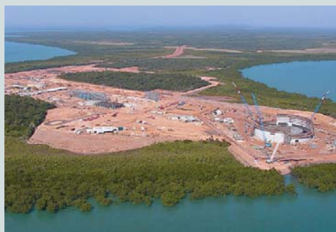
Construction of the Darwin LNG facility in Australia.
